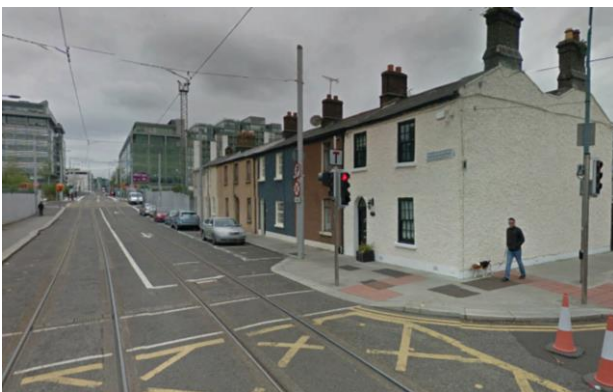
Photo 3: View of existing residential dwellings to the front of site along Mayor Street Upper
