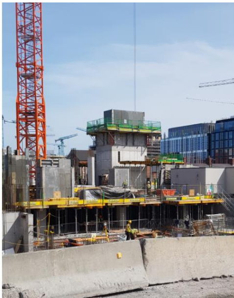
Photo 8: Construction Progress on site
