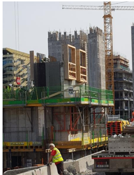
Photo 9: Construction Progress on site
