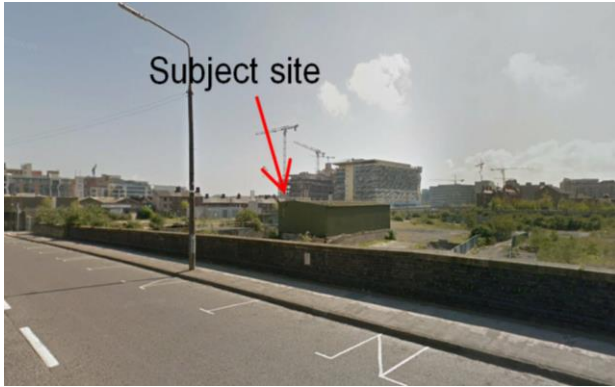
Photo 6: View of site from Sherriff Street Upper
